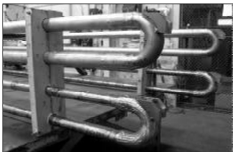
Completed USC test loops (shown above) prior to being delivered to the Niles plant for installation
