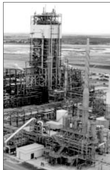
TECO's 250-MWe Polk Power Station, Unit 1 IGCC facility
