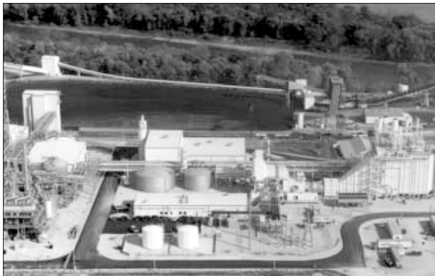
Wabash River Generating Station repowered with a 262-MWe IGCC unit
