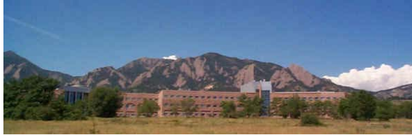
David Skaggs Research Center, Boulder, Colorado, USA
