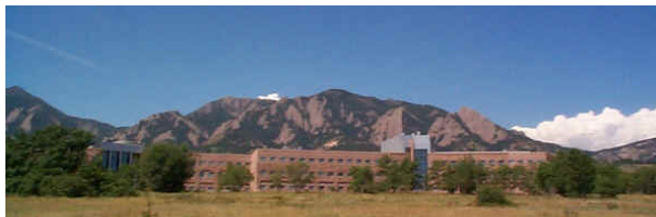
David Skaggs Research Center, Boulder, Colorado, USA
