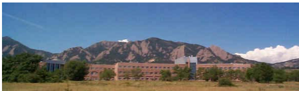
David Skaggs Research Center, Boulder, Colorado, USA
