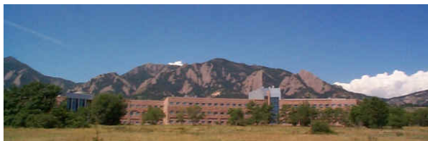
David Skaggs Research Center, Boulder, Colorado, USA
