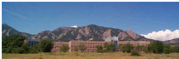
David Skaggs Research Center, Boulder, Colorado, USA
