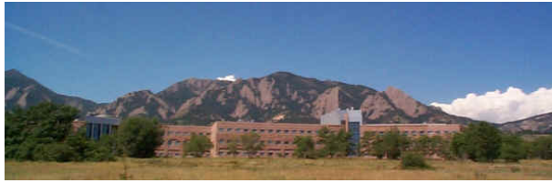
David Skaggs Research Center, Boulder, Colorado, USA
