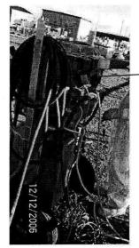
Three unused extension cords left plugged into the portable power panel.
