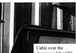
Cable over the doorway of the C91 Building showing wear from the rain lip edge.
