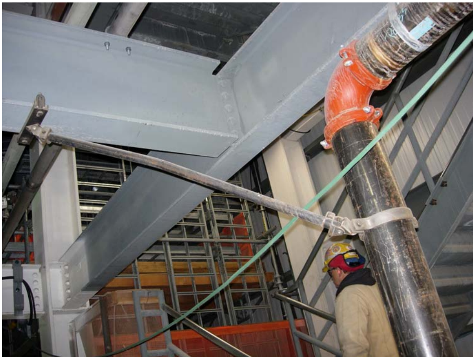
Figure 2: Bent Sway Bracing on North East +28 elevation
