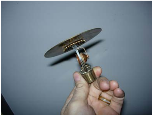
Figures 8 and 9: Example intermediate level sprinkler head (left) and sprinkler head guard (right)
