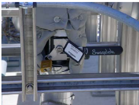
AN Demister Valve and Lock
