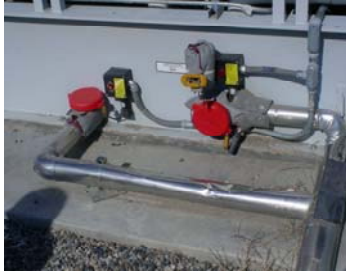
AW Seal Pot Drain Valve Locks
