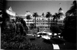
The Hotel Del Coronado is within a RDA project area.
