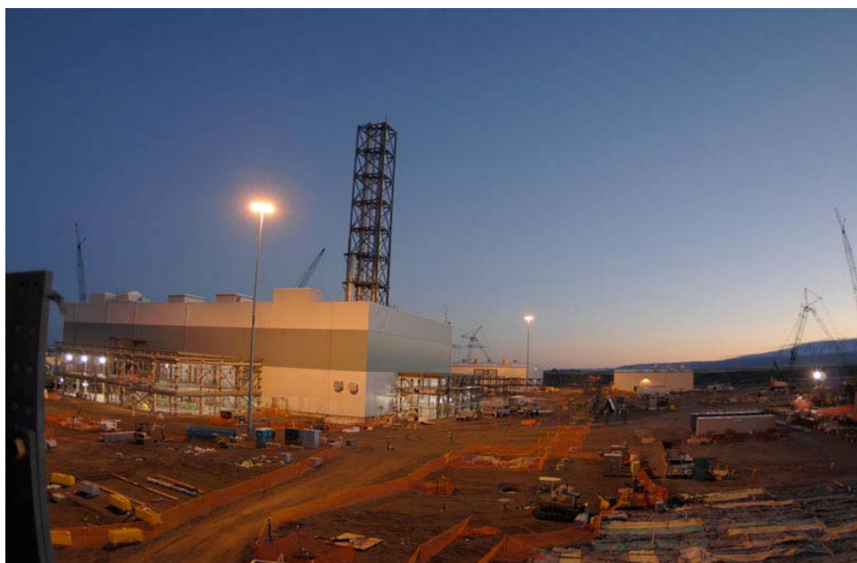
Figure 1. Low-Activity Waste Facility – as seen from the PT Facility
