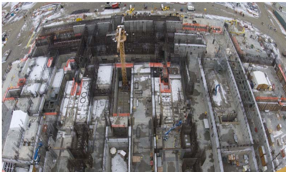
Figure 4. High-Level Waste Facility – as seen from the Tower Crane
