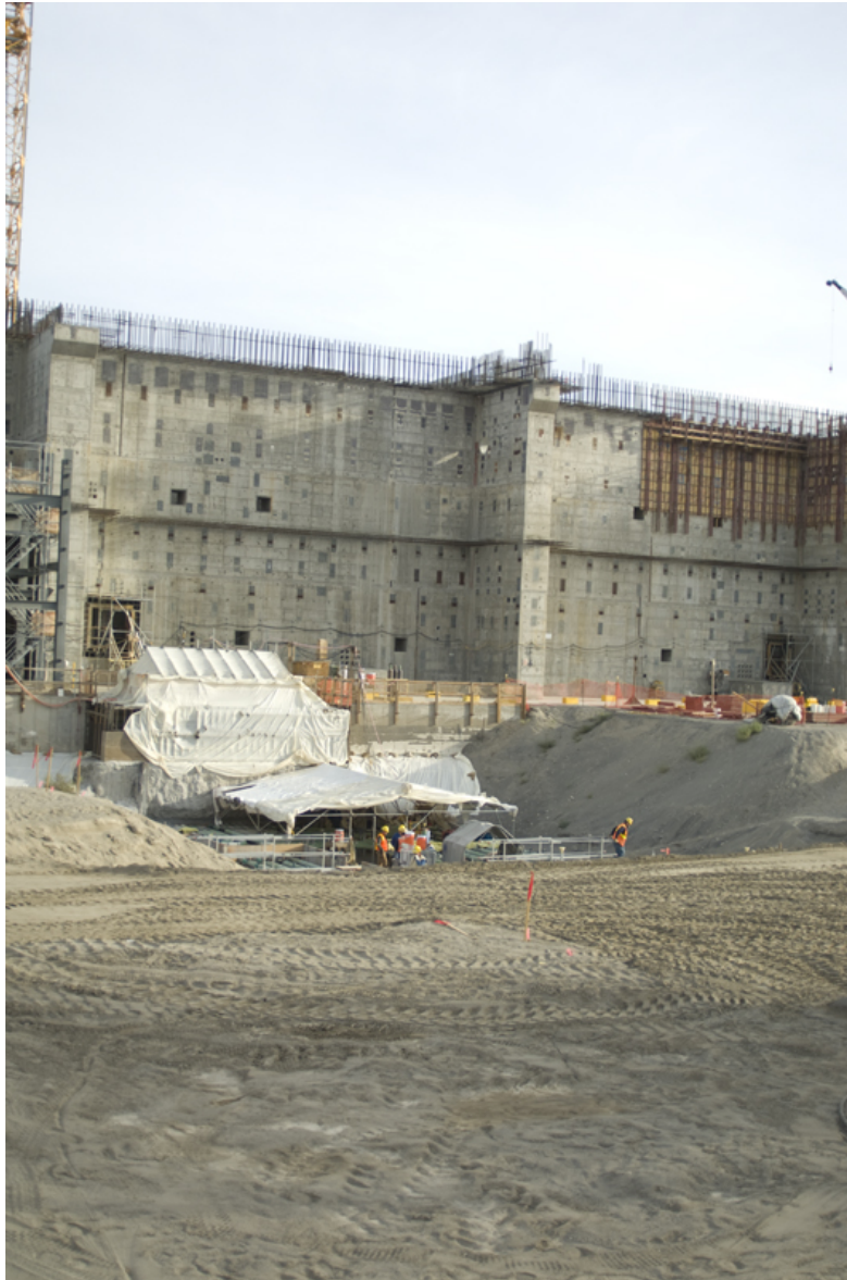
Figure 10. Excavation Work near Pretreatment Facility
