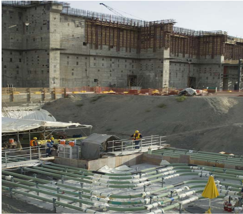
Figure 11. Pretreatment Facility – Southside Transfer Line Work
