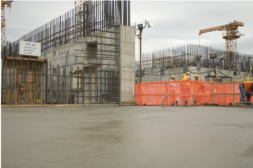
Figure 8. High-Level Waste Facility – Complete Slab at Southwest Corner
