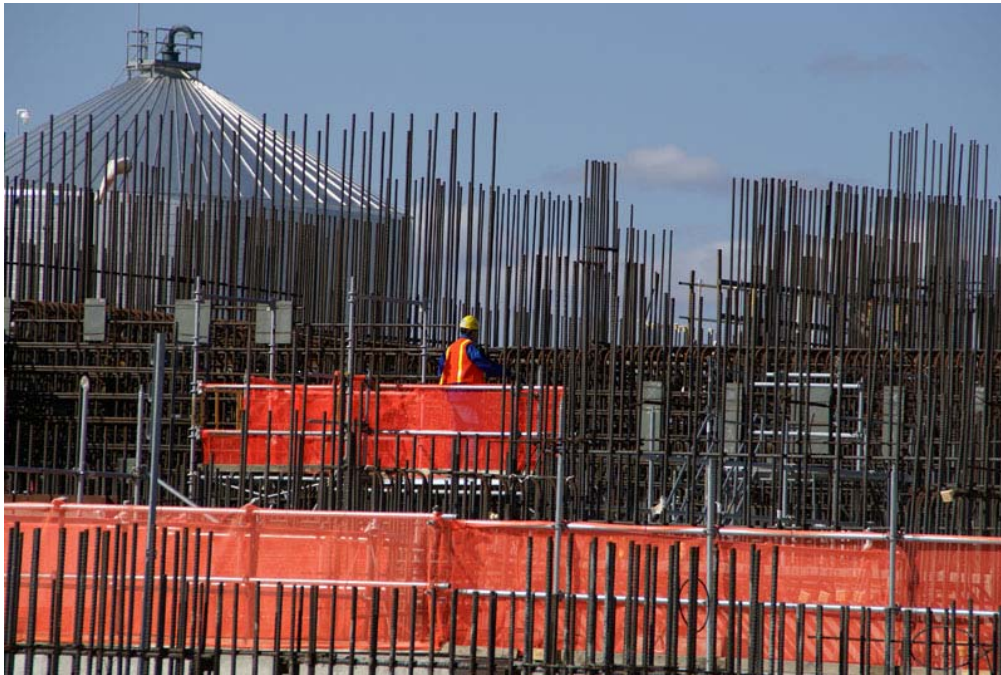
Figure 9. High-Level Waste Facility – Rebar on East Side
