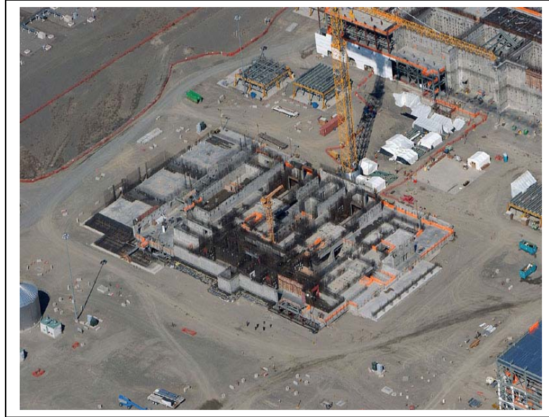
Figure 5. High-Level Waste Facility
