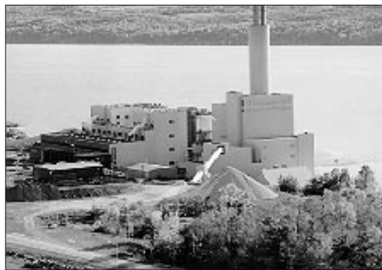
The combined \text{SO}_2/\text{NO}_x control process demonstration at the 300-MWe Milliken Station (two 150-MWe tangentially-fired units) began in January 1995.
