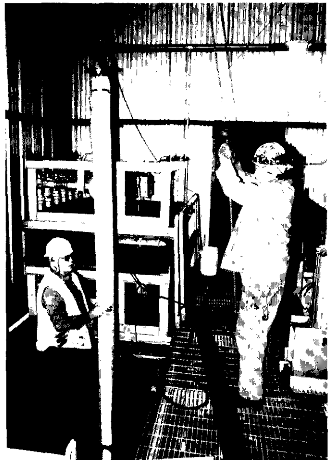
Nextel Bag Assembly Containing SCR Catalyst is Lowered Into Baghouse Module Tubesheet
