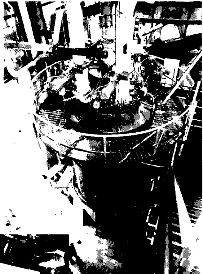
Left: Coal Reburn Burners Installed During Fall 1991 Outage. Photo shows One of the Four Burners Being Installed, and a Port to the Left Being Prepared for Burner Installation. Wisconsin Power & Light Nelson Dewey Station Unit No. 2, Cassville, WI. 100 MWe.
