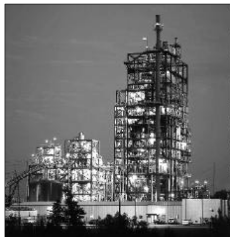
The Power Systems Development Facility as seen at night
