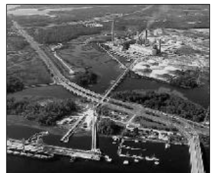
Aerial views of JEA plant
