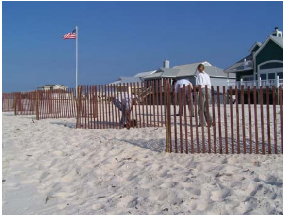
Fig. 5. Sand fence installation where turtle nesting is a concern.
