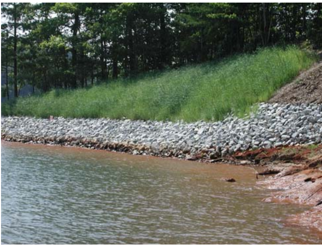
Streambank Stabilization (Alamo switchgrass)
