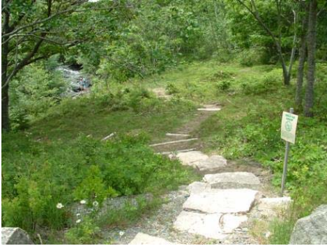
Stabilizing a steep trail path
