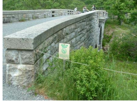
Stabilizing a steep slope along Carriage Road Bridge
