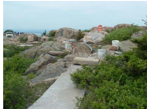
Trail construction on Cadillac Mountain
