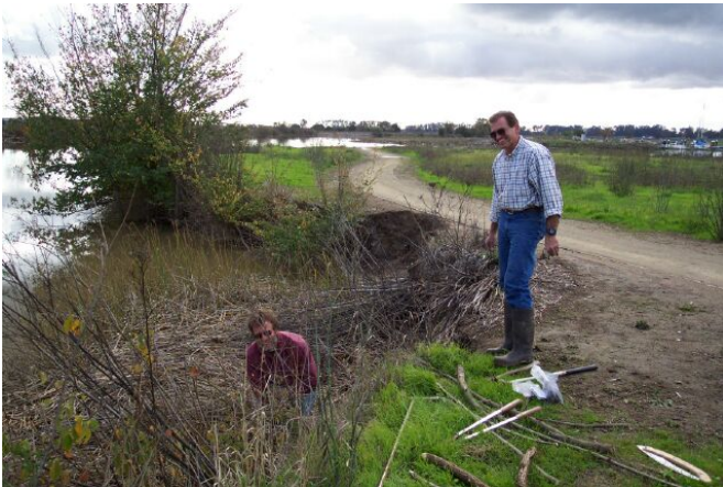
Willow cutting being driven into stream bank at Huichica Creek
