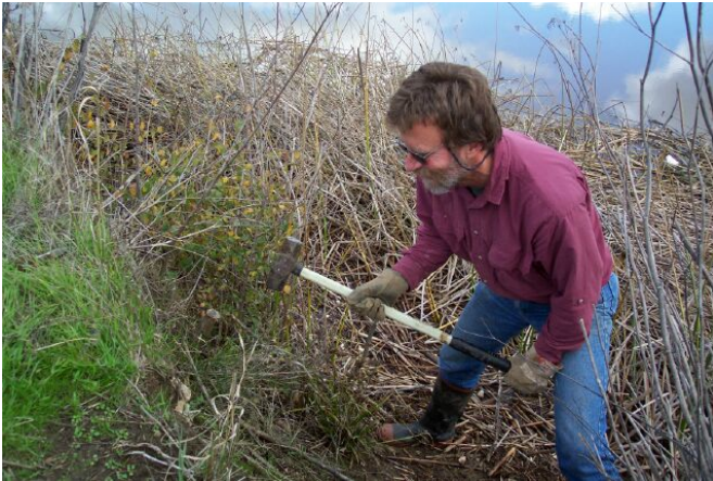
Willow cutting being driven into stream bank at Huichica Creek
