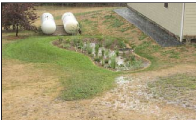
Figure 2. A new rain garden captures roof and yard runoff from a ½ inch, 15-minute prairie thunderstorm in July. Note the drought stressed yard outside the rain garden.
