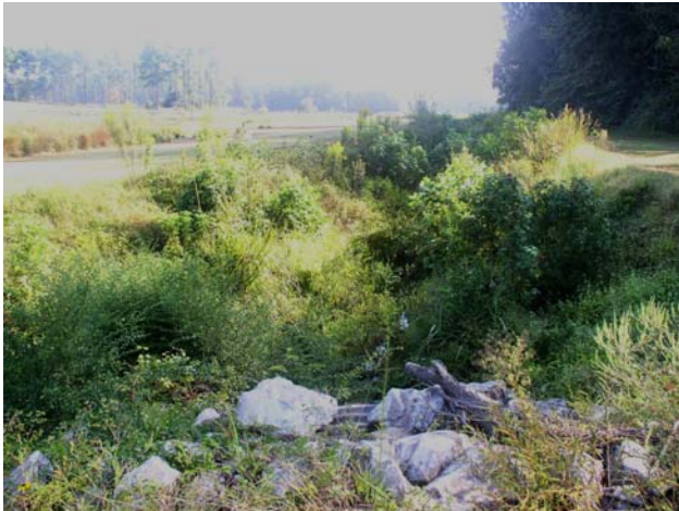
Ditch before repairs
