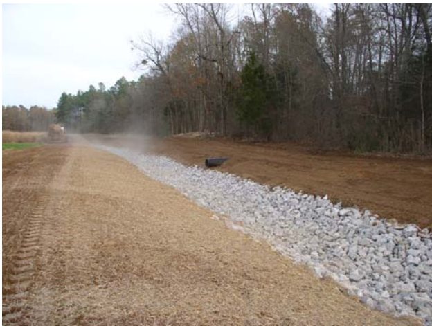
Ditch after repairs
