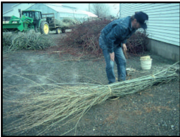
Preparing live fascines for planting
