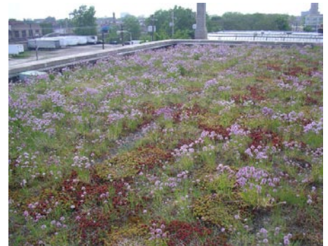
E11 Green roofs help stabilize building temperatures and reduce stormwater runoff
