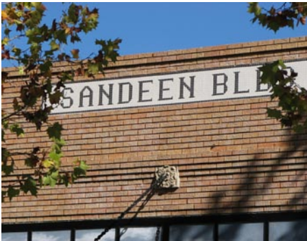
Brick and stone are common building materials
