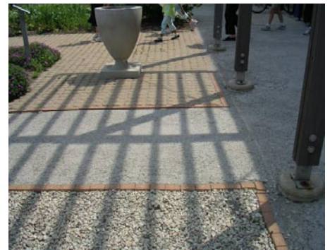
E13 Permeable pavers absorb runoff and provide alternate paving materials that can add identity to a streetscape
