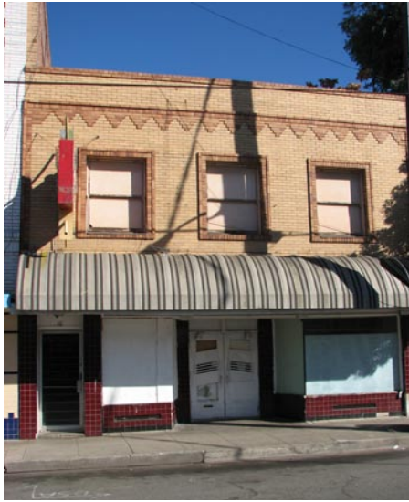
Boarded up building east of the tracks
