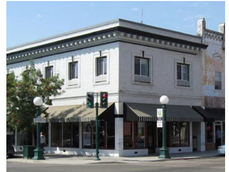
B4 Successful adaptive reuse of upper floors
