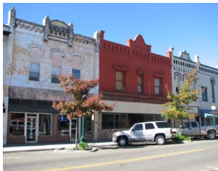
Facade restoration along historic buildings on Sacramento Street
