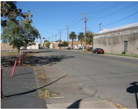
Lack of sidewalks, curb and gutter along Main Street
