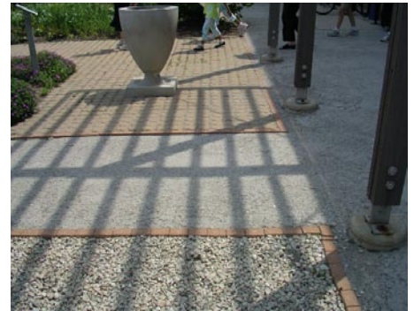
E13 Permeable pavers absorb runoff and provide alternate paving materials that can add identity to a streetscape
