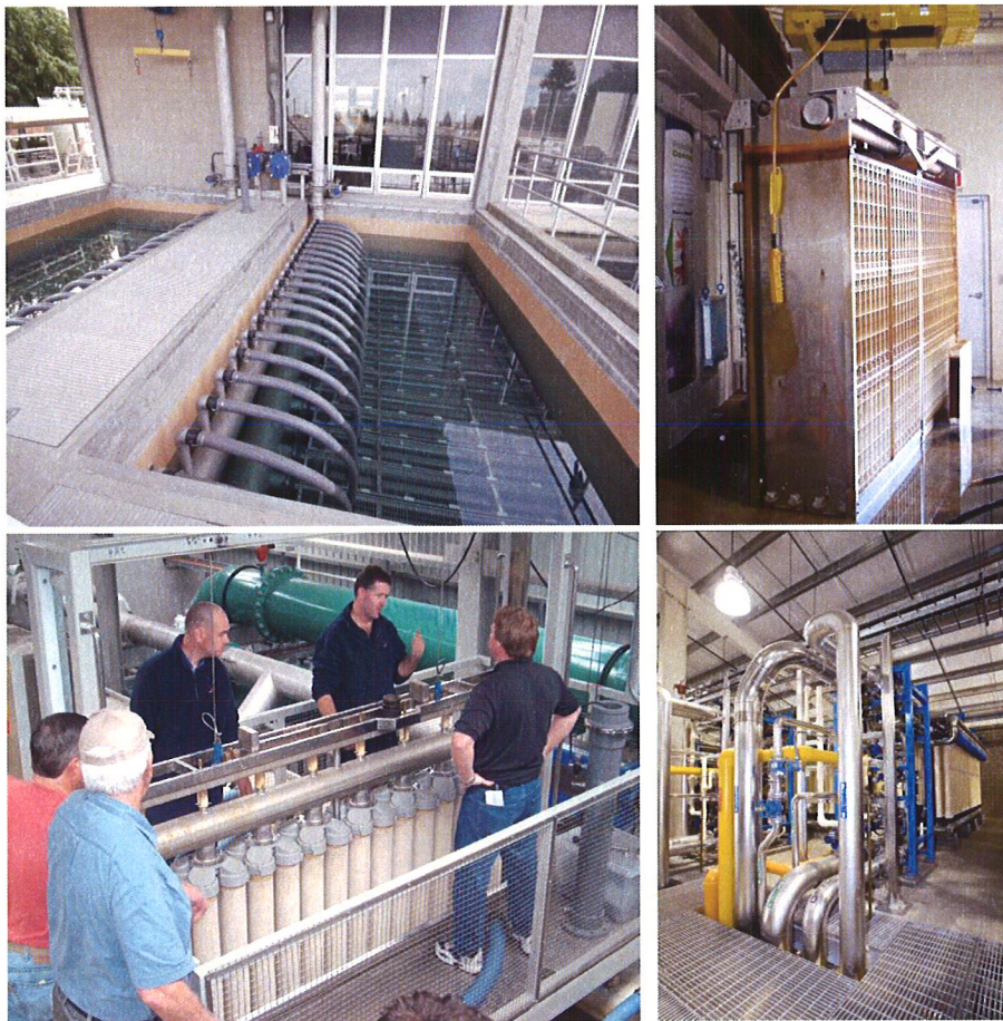
Picture of two Memcor submerged membrane systems (Yuba City, CA- upper left, and Bendigo, Australia- lower left), a Zenon 1000 membrane cassette module (South San Joaquin Irrigation District-upper right), and a Pall pressure membrane system (Yucaipa Valley Water District- lower right)
