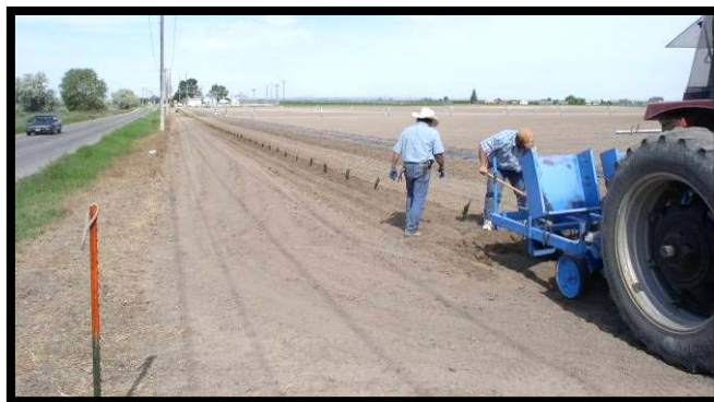
Installing new Rocky Mountain juniper and Simon poplar windbreak
