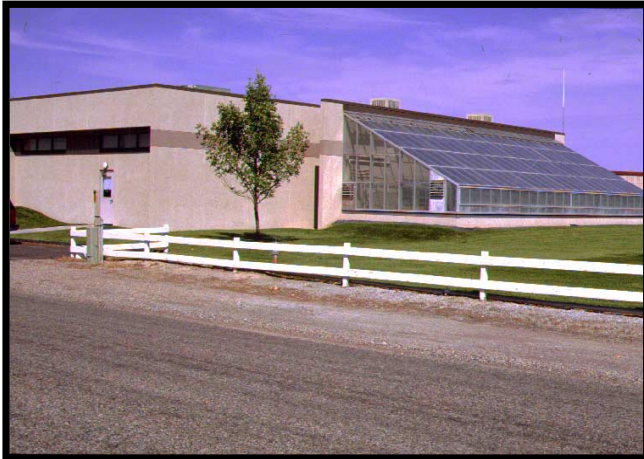
Aberdeen Plant Materials Center office and greenhouse
