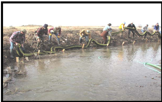
AZ workshop participants laying out a new organic soil filled sock that could either replace a willow fascine or added to it for more protection.
