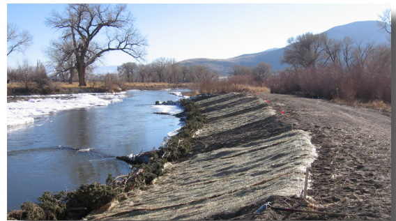
Erosion control netting was placed on streambank to test seedling growth.
