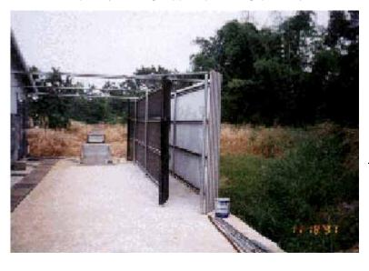
exhaust fans are diverted upward. This effect promotes mixing of the odorous, dusty airflow with the wind passing over the building, so that the plumes of air pollutants originating from the fans are made larger (extend higher) in addition to the physical trapping of odor particles on the windbreak.
