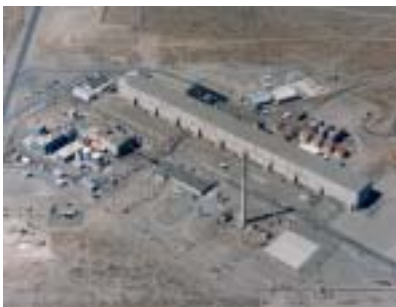
Exterior view of U Plant, one of five massive fuel separation facilities, also known as canyons, on the Hanford Site.
