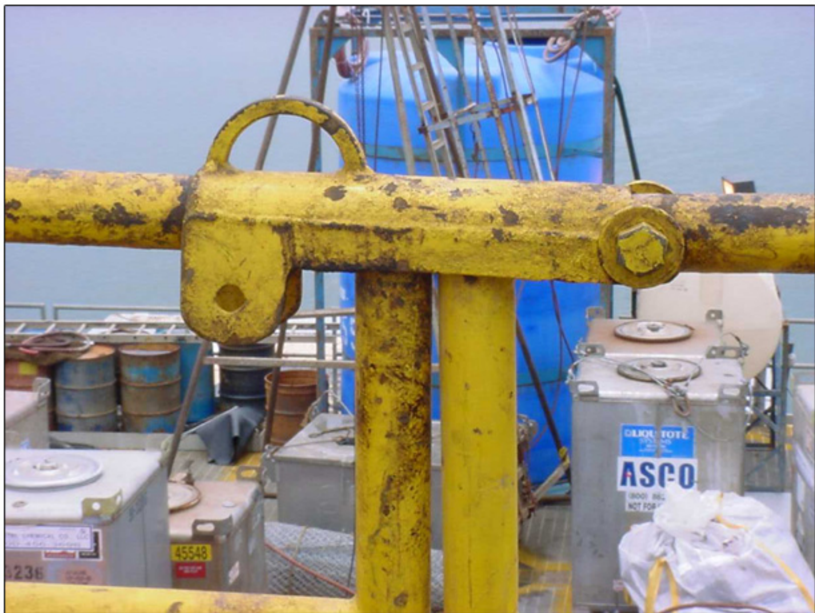
Close View, Gate Fastener and Lock Hole
