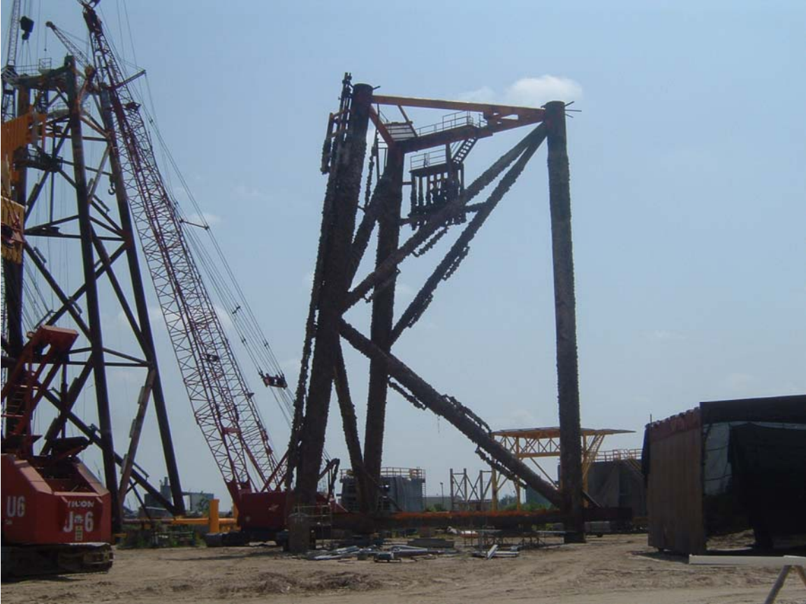
Figure C.15. Jacket Structure in Storage at Unifab’s Facility in New Iberia, Louisiana-I.
