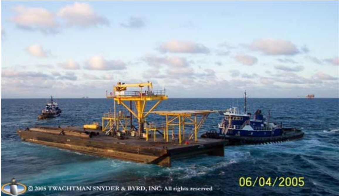
Figure C.5. Deck Module and Heliport Transported to Shore (Twachtman Snyder & Byrd, Inc., 2006).
