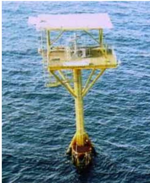
Figure E.1. Caisson Structure in the Gulf of Mexico (Twachtman Snyder and Byrd, Inc., 2006).
