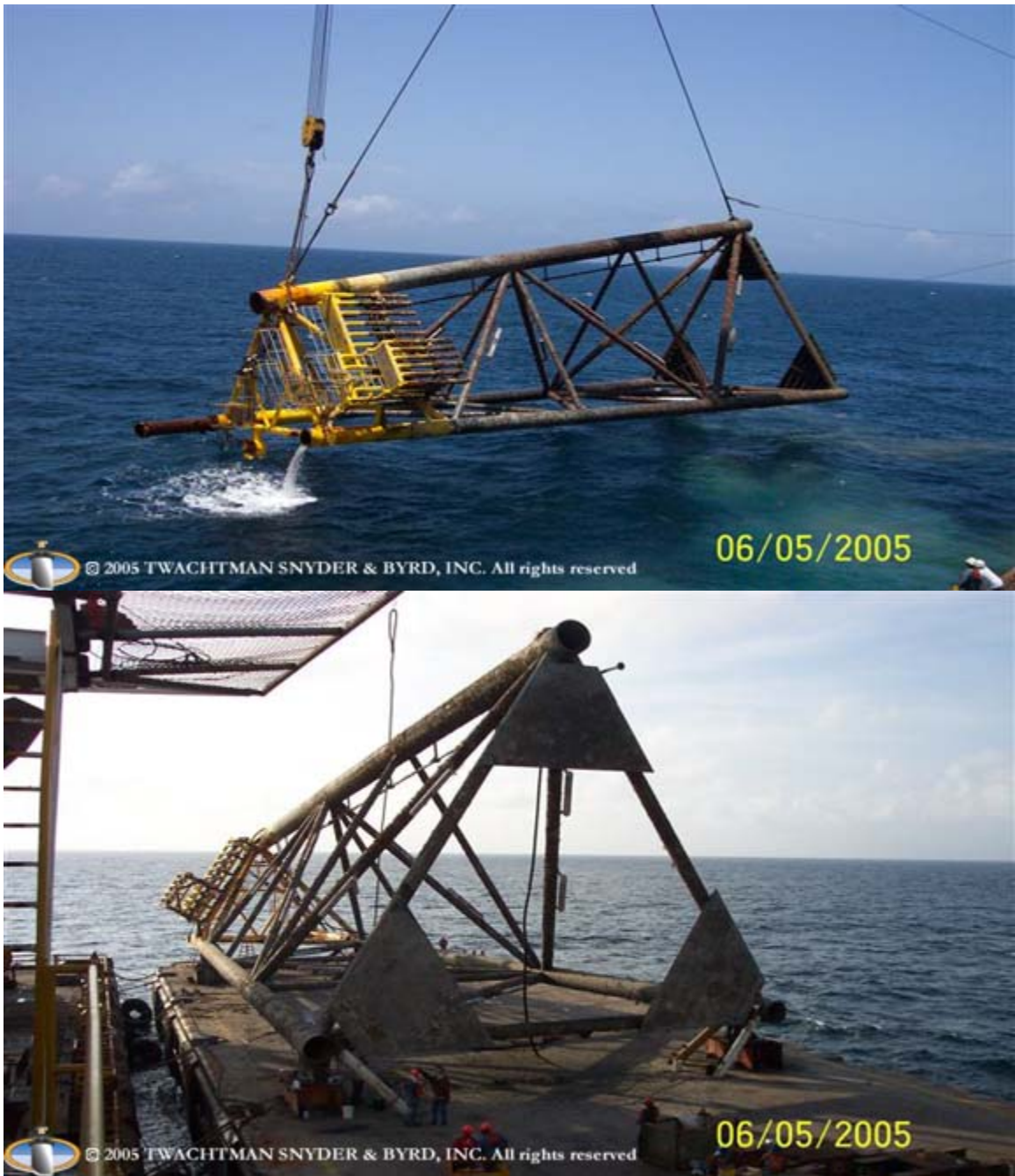
Figure C.8. Jacket Lifted from Water and Transported to Shore or Artificial Reef Site (Twachtman Snyder & Byrd, Inc., 2006).
