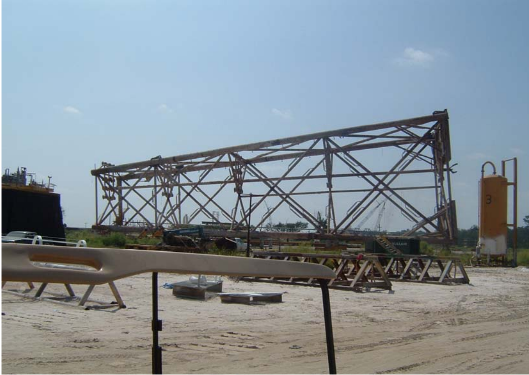
Figure C.14. Jacket Structures Stored Onshore Awaiting Dismantlement or Reuse Opportunity.
