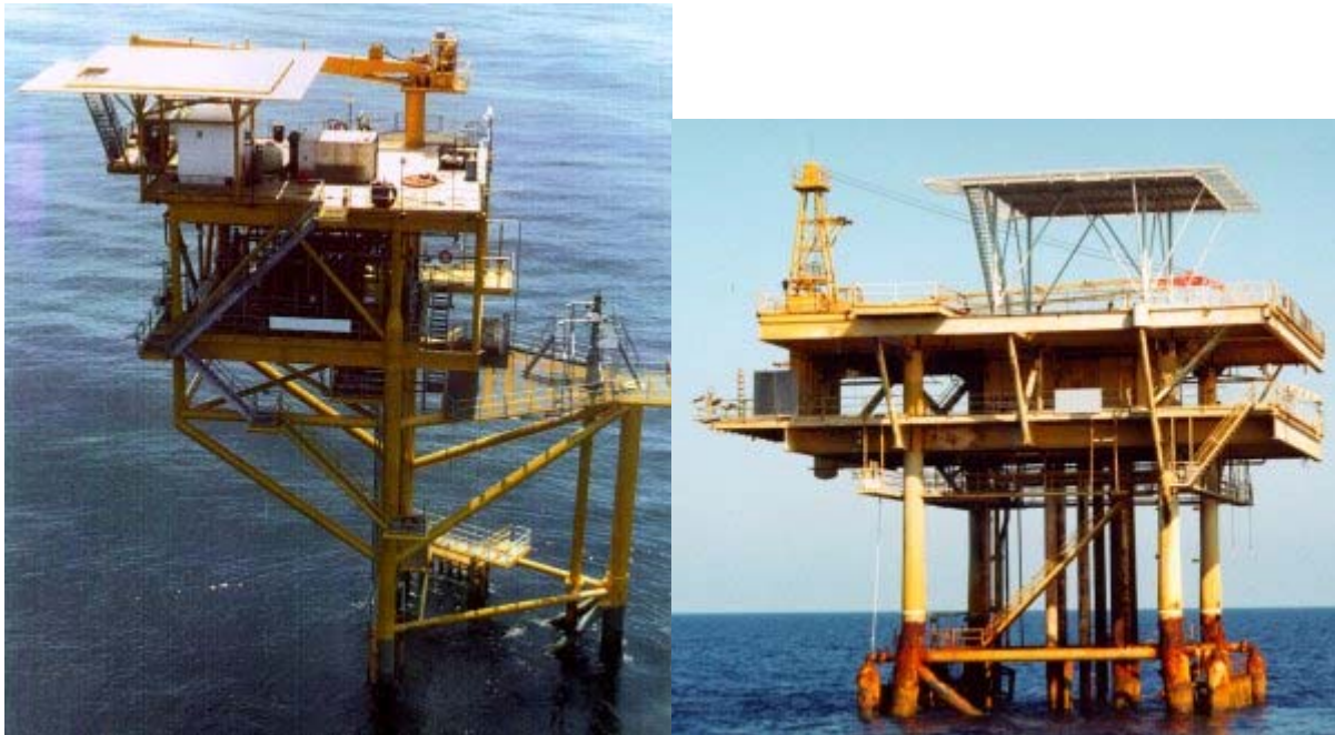
Figure E.2. Well Protector Structures in the Gulf of Mexico (Twachtman Snyder and Byrd, Inc., 2006).
