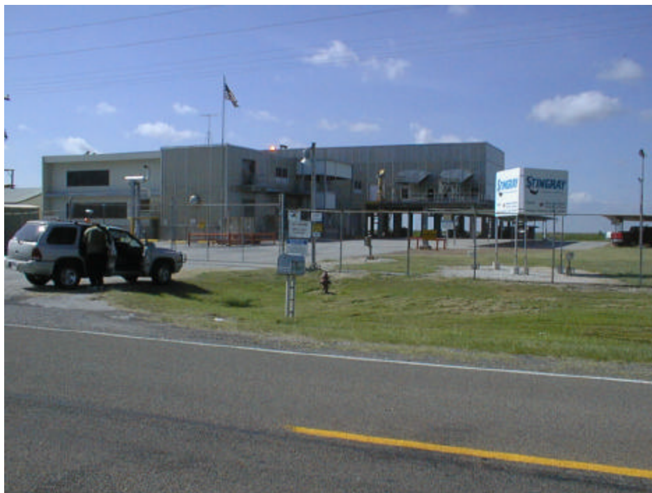
Figure 3.2 Determining Geographic Position of a Pipeline Facility with GPS
