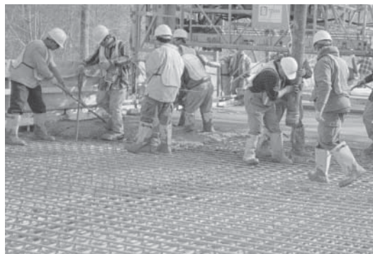
Workers place high-performance concrete on a new bridge in a national park.
