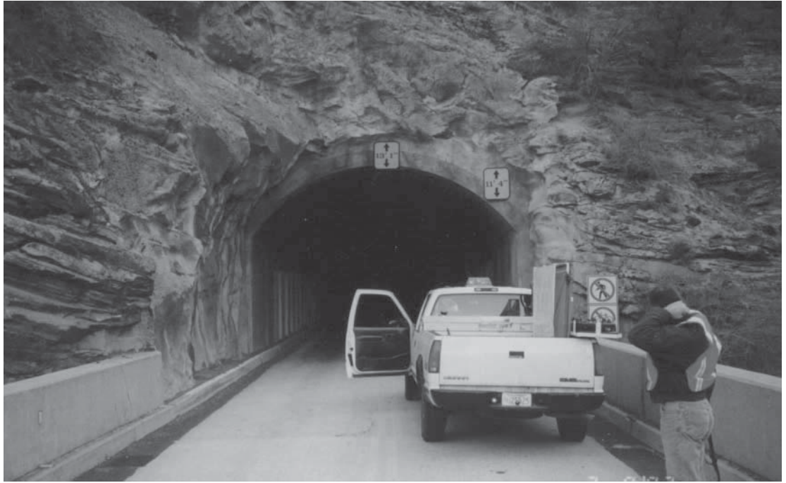
Entrance to the Zion–Mt. Carmel Tunnel, Zion National Park, Utah. Inside the tunnel, FHWA staff use True Reflection Tomography™ to assess the technical and economic feasibility of enlarging the tunnel.
