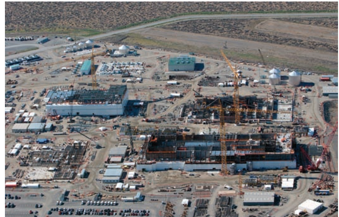
Construction of the Hanford Waste Treatment Plant in Washington State.
