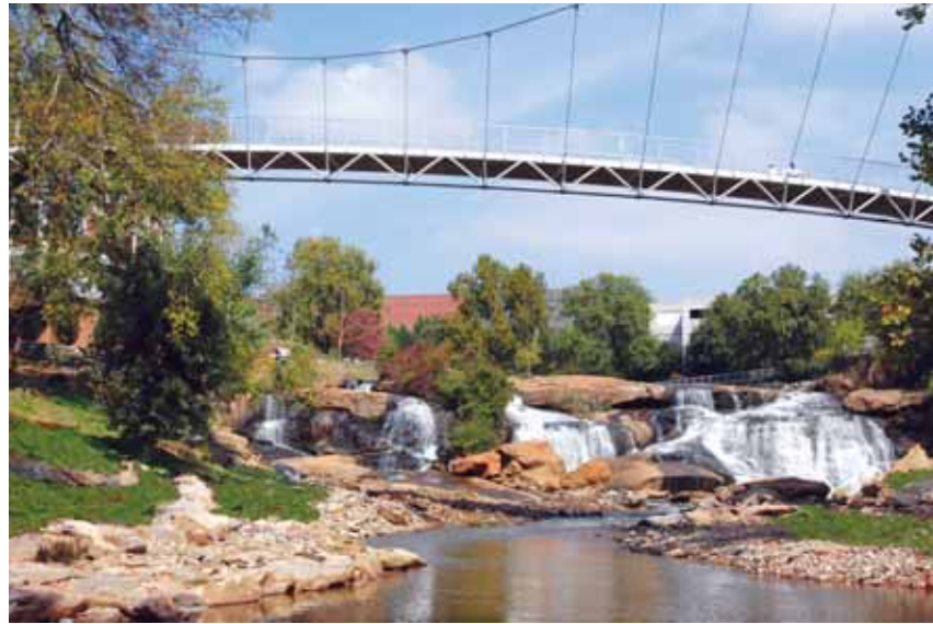
A vehicular bridge that once obstructed this waterfall was replaced by this pedestrian bridge. The project was part of a park renovation that took place when the Peace Center for the Performing Arts was developed.
