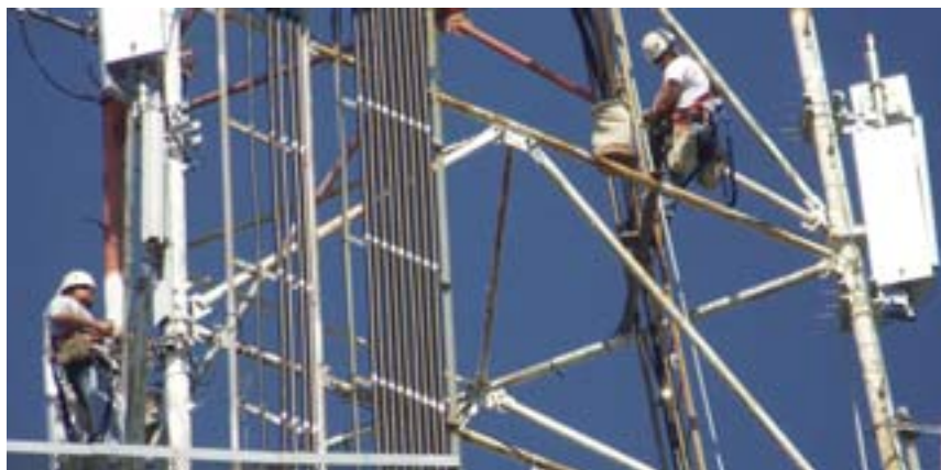
Technicians install antennae on existing towers throughout the GRADD region, which will bring high-speed wireless Internet service to residents of the predominantly rural region.
