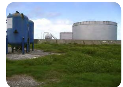
Old fuel tanks located in "no-dig" area
