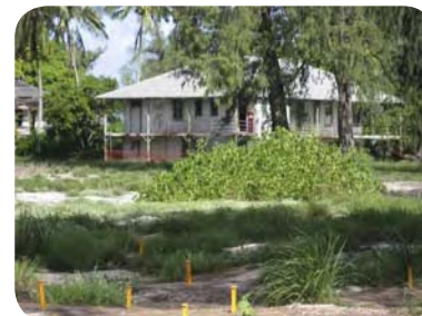
Cable Station building complex
