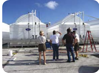
New fuel tanks lead industry in spill protection
