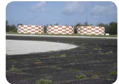
Water collection tanks
