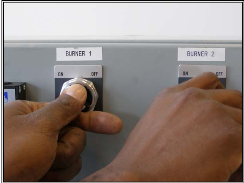
Figure 3. Step 9 Turn burner switches to "ON" position.
