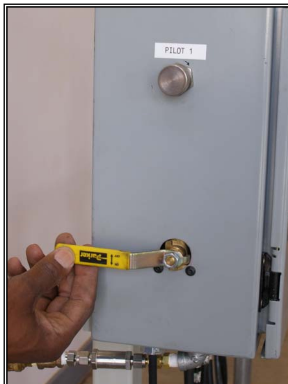
Figure 31. Step 32 Open pilot ball valves.
