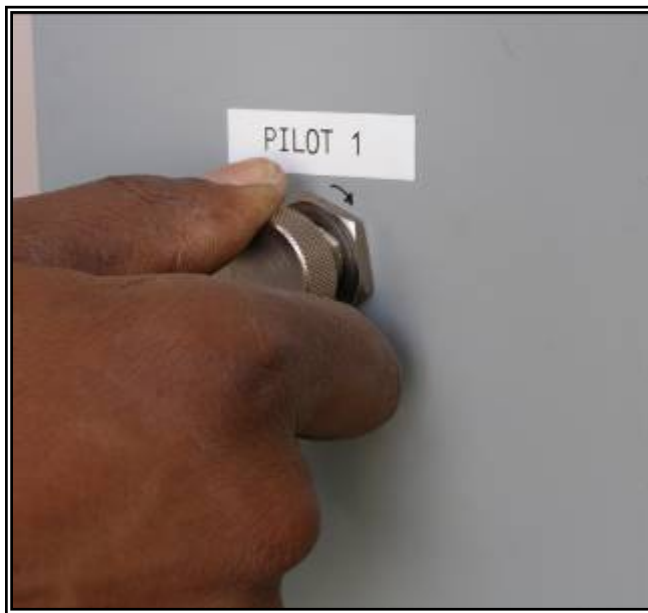
Figure 12. Step 10 Set pilot flow.
