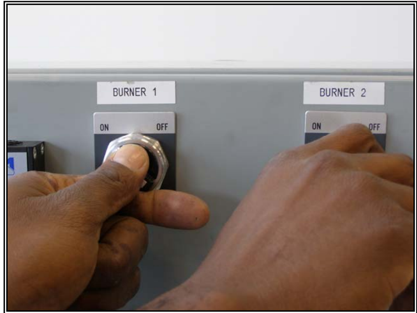
Figure 33. Step 37 Turn burner switches to "ON" position.
