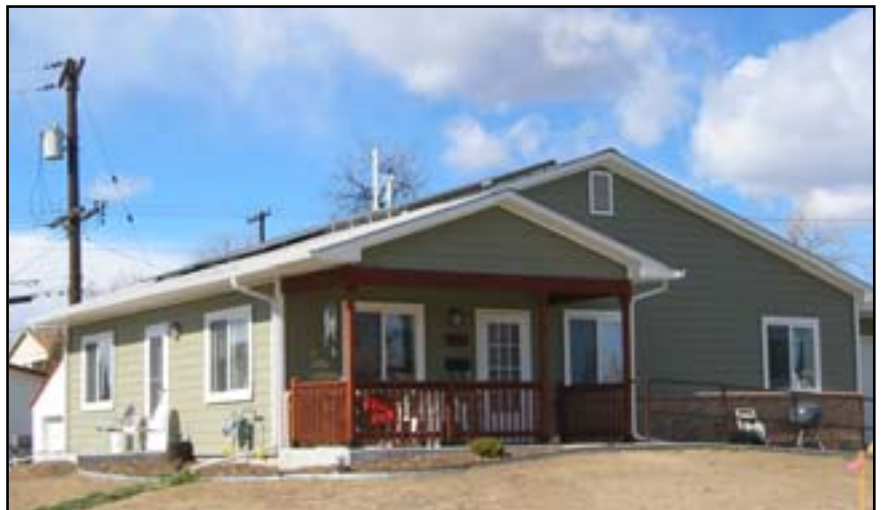
Habitat Metro Denver used Building America's integrated design approach to build this award-winning home in Denver, Colorado.
