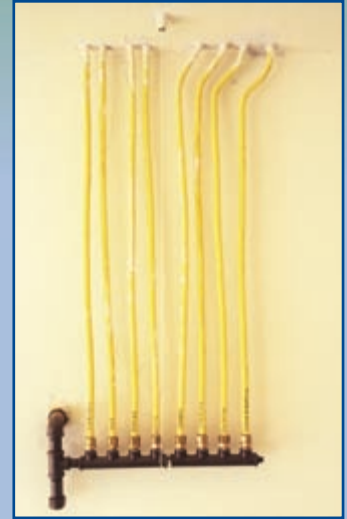
This manifold piping distribution system is easier to install than traditional systems.
