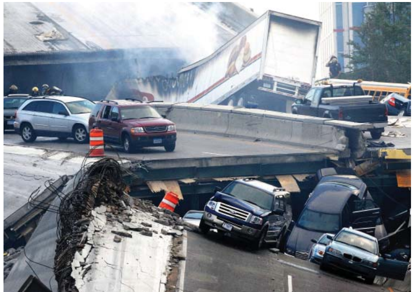
Vehicles are scattered along the broken remains of the Interstate 35W bridge, which stretches between Minneapolis and St. Paul, after it collapsed into the Mississippi River during evening rush hour Wednesday, Aug. 1, 2007, sending vehicles, tons of concrete and twisted metal crashing into the water. (AP Photo/The Minnesota Daily, Stacy Bengs)
