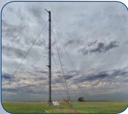
The SGP site in Oklahoma provides a wide variability of climate cloud types and surface flux properties, and large seasonal variation in temperature and specific humidity.
