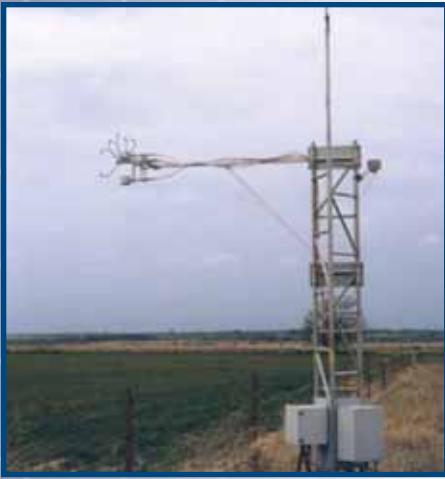
The new ECOR systems use proven technology selected on the basis of successful deployments of similar systems at SGP by other organizations.
