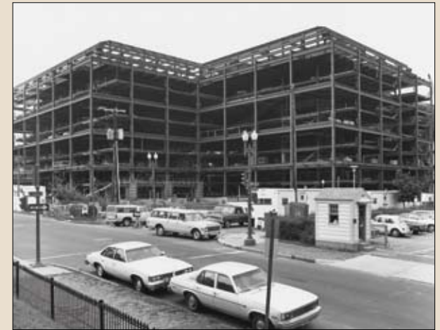
Hart Senate Office Building under construction.
