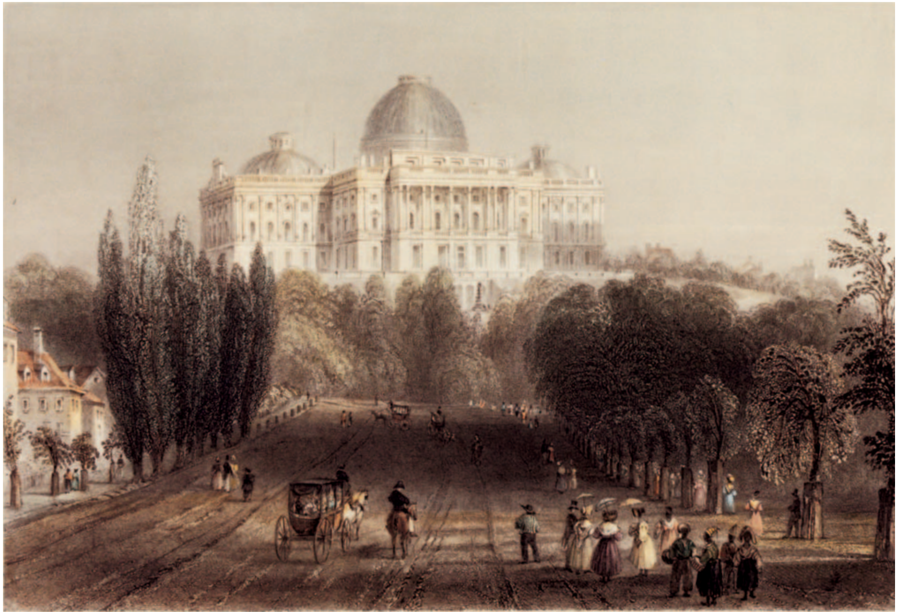
NORTHWEST VIEW OF CAPITOL 1840.
